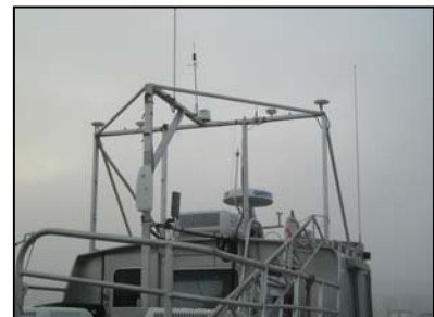
Antenna Mast Configuration
